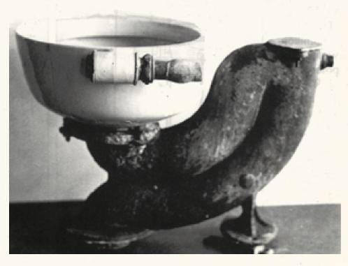
ers to follow Cummings lead. Two years later in 1777, Samuel Prosser applied for and received a patent for a plunger closet. On his heels came Joseph Bramah, only one year later. His closet had a valve at the bottom of the bowl that worked on a hinge—a predecessor to the modern ballcock. Himself a bit of a sailor, Bramah's closet was used extensively on ships and boats of the era.
